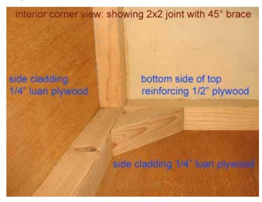
The photo at left shows the insidetop-corner view of a typical pedestal.
